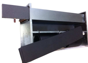
Retirer le bloc mousse anti- condensation
